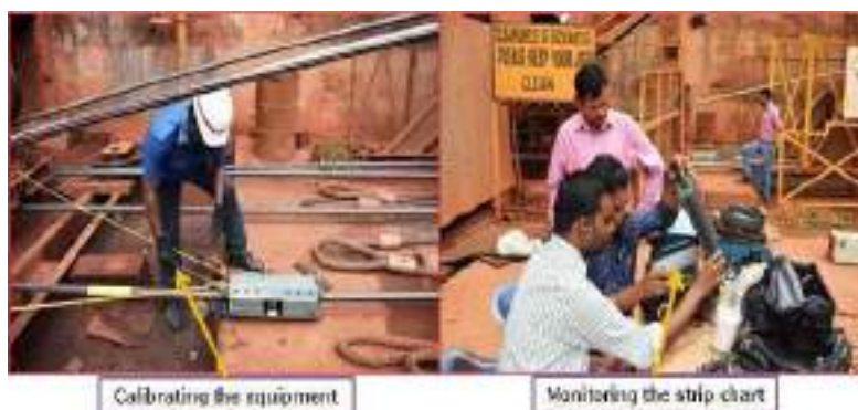
Inspection of Left side rope
