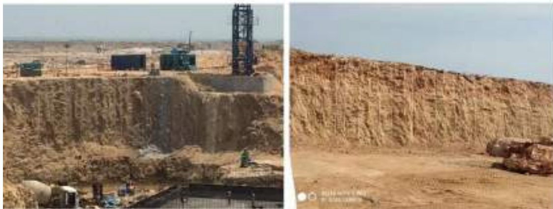
Controlled blasting close to green concrete
