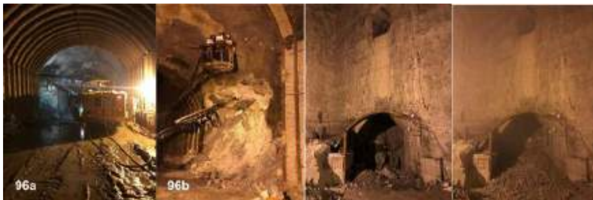
Excavation of expansion chambers at Punatsangchhu II Hydroelectric Project
