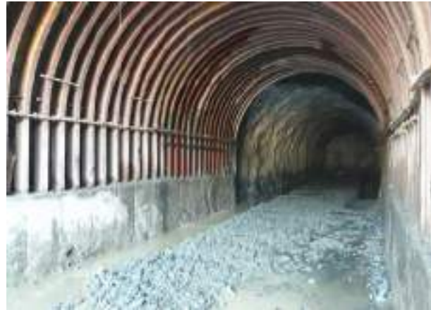
A view of completed D shape portion of pressure shaft from powerhouse
