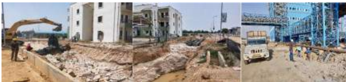
Controlled blasting near field hostel for sewerage line, close to the permanent structures of NTPC at Darlipalli STPP
