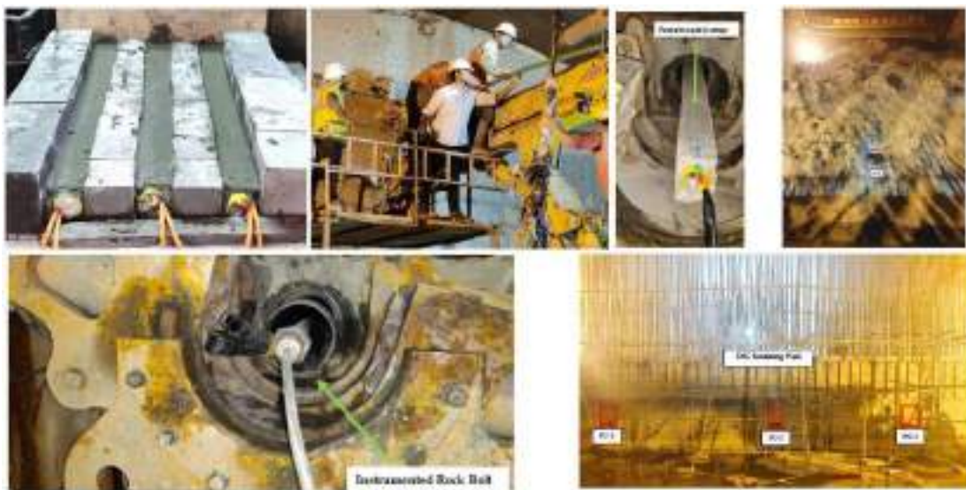
Installation of prefabricated setup comprising of load cell and biaxial borehole stress meter, Instrumented Rock Bolt in fallen muck and pressure cells to monitor lateral thrust on the retaining walls of DSC
