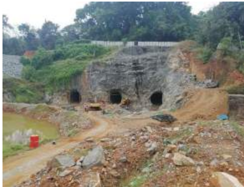
Excavation of 3 tunnels near Pazhassi Sagar barrage
