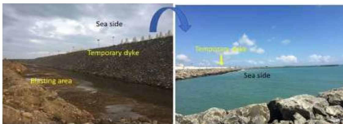
Controlled blasting close to a temporary dyke
