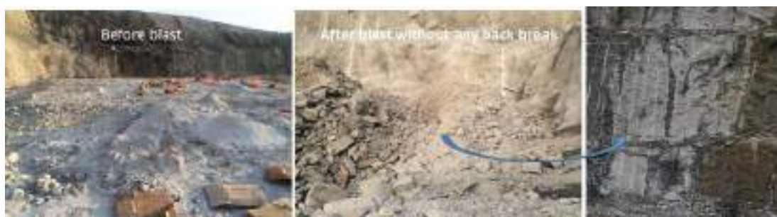
Slope obtained as a result of presplit blast design
