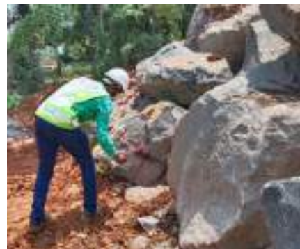
Marking of armour rock at stock pile.
