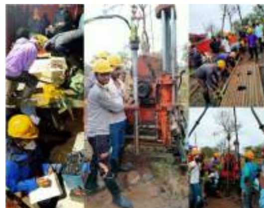
Goodman Jack test in progress at BH-18
