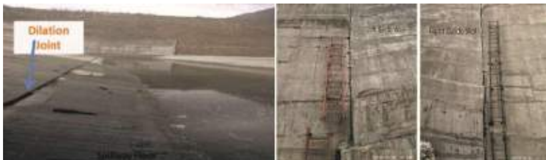
Visual damage seen around flip-bucket (left) and widening of joints on guide-wall (right)
