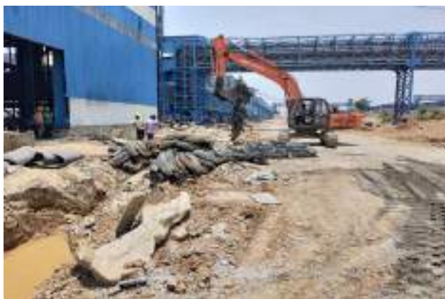
Controlled blasting adjacent to the structures
