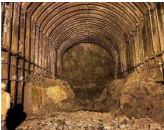
Final benching excavation in AST-N1a at RD 110
