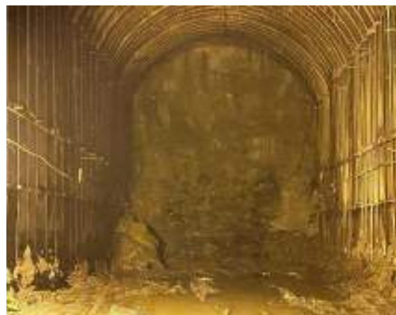
Final benching excavation in AST-N1a at RD 110
