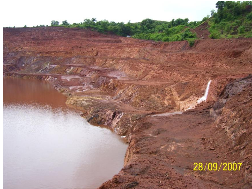
Fig. 8.3 Water seepage within the pit slopes at an iron ore mine in Goa
