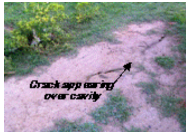
Fig. 2.5 Surface crack seen above cavity pocket
