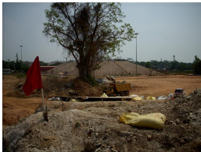
Fig. 7.7 Preparation of blasting near bullet tank area
