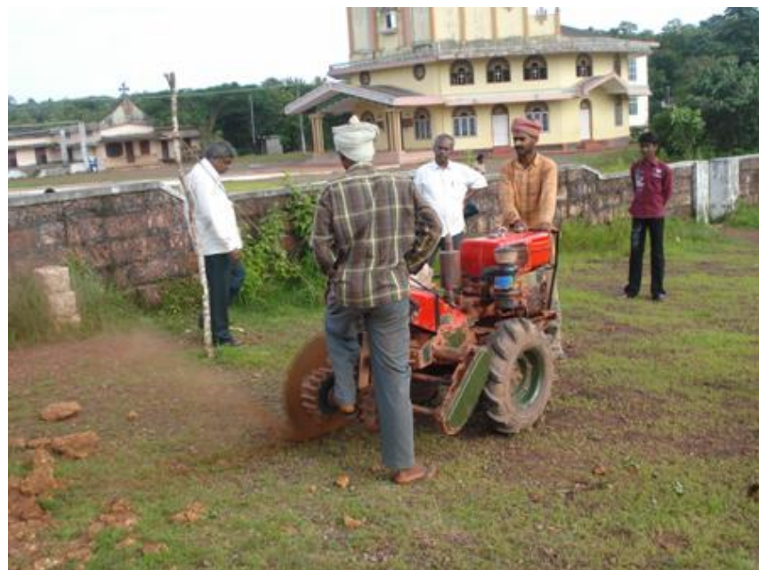
Fig. 9.2 Rock sample being extracted using laterite cutting machine
