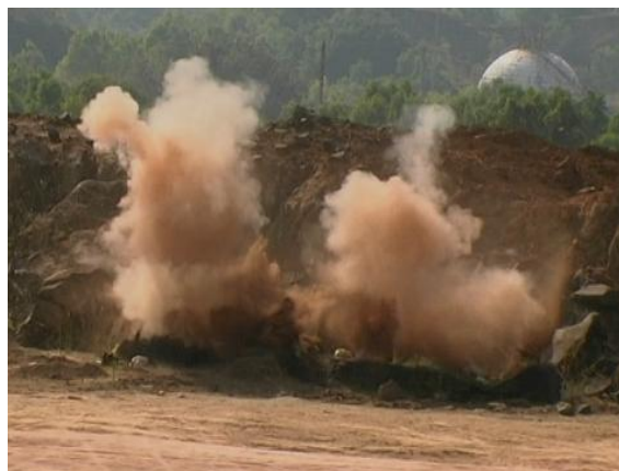
Fig. 7.4 Blasting near storage tanks
