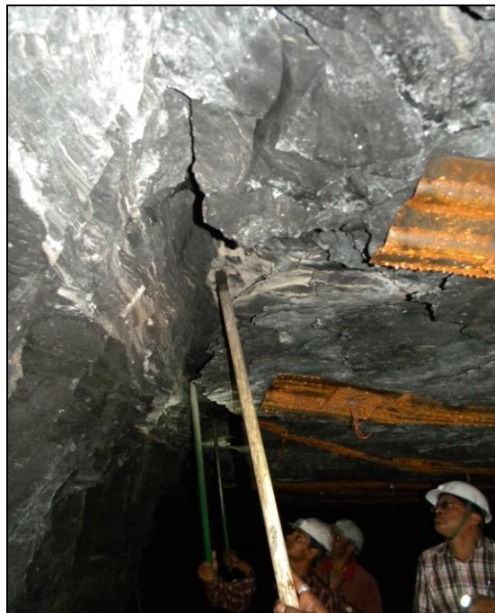
Fig. 8.2 Bad roof conditions experienced at Mathani mine, WCL
