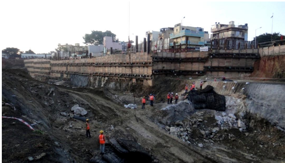
Fig. 7.6 Controlled blasting at City railway station area
