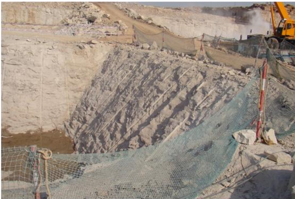
Fig. 7.1 Good pre-split blast result in hard rock in slopes
