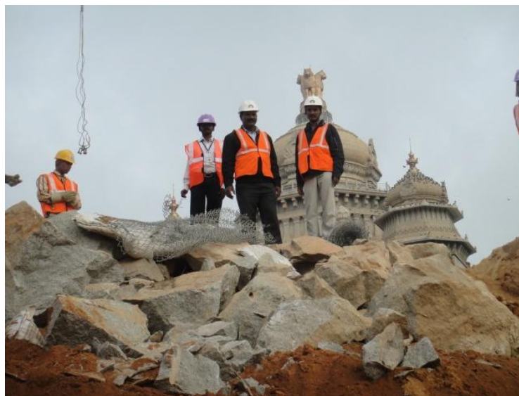
Fig. 7.5 Post-blast inspection of the blast area near Vidhana Soudha by NIRM
