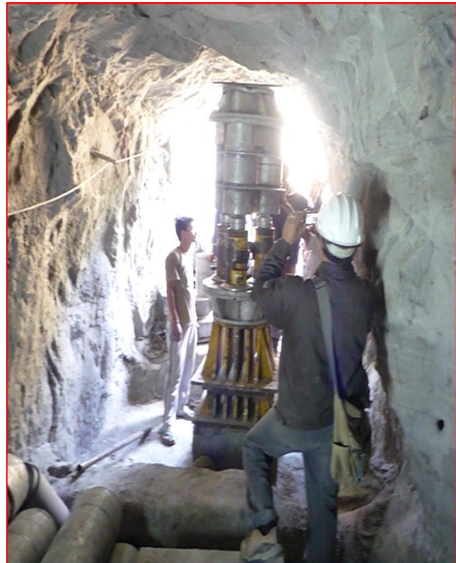
Fig. 3.2 Direct shear test set-up at the test site
