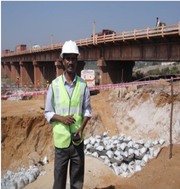
Fig. 7.8 Muffled block ready for blast adjacent to the existing bridge
