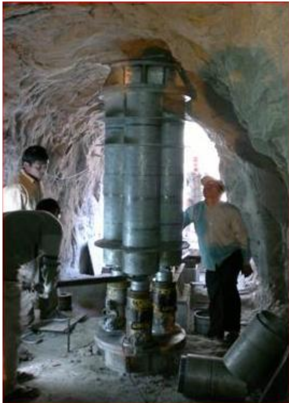
Fig. 3.1 Plate load equipment set-up at the site
