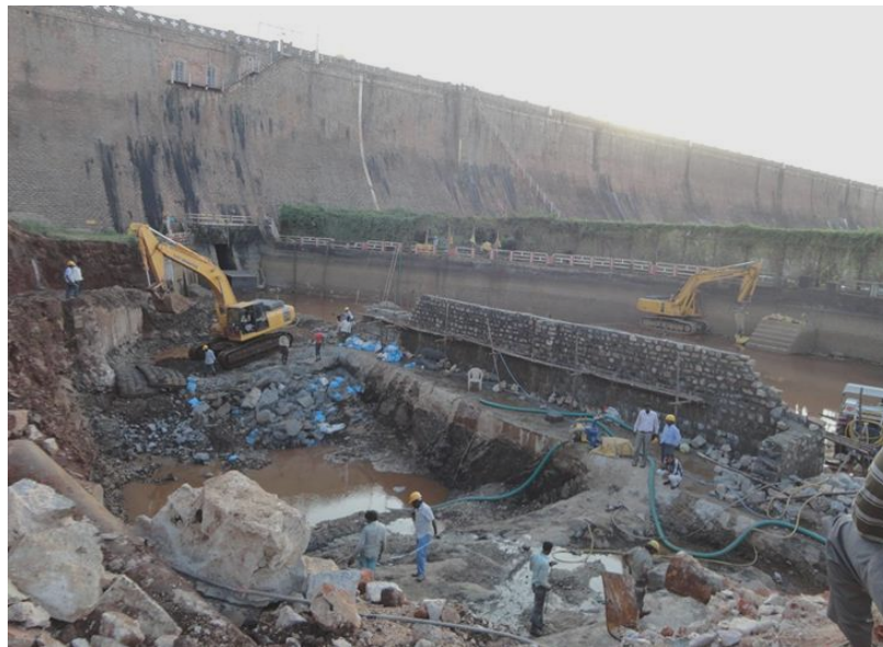
Fig. 6.1 Controlled blasting activities close to Tunga Bhadra dam and canal
