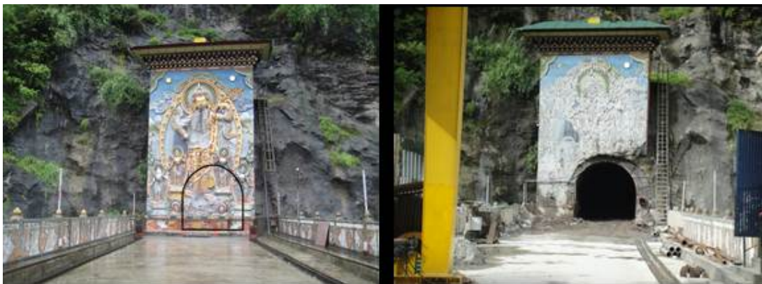
Fig. 6.2 Location of adit portal, and the excavated adit along the axis of Tala dam, Bhutan
