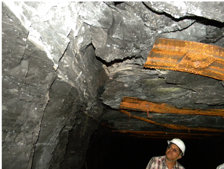
Fig. 7.1 Cutter roof conditions at Mathani colliery
