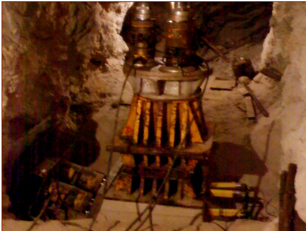
Fig. 3.2 In-situ shear investigations inside the drift at left bank of dam site at Mangdechhu HE Project
