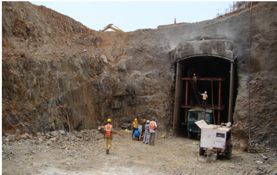
Fig. 1.1 Center heading method for north RHS portal area of Hungund-Hospet road tunnel showing jointed and moderately weathered metabasic rock
