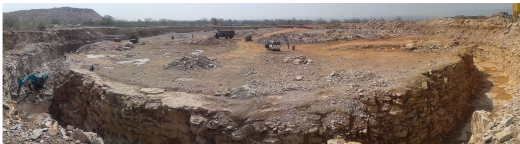
Fig. 1.7 Foundation level of NDCT-8A of RAPP Unit 8
