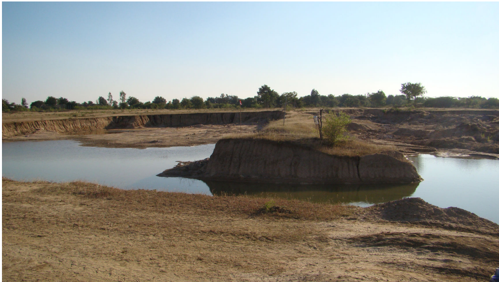
Fig. 1.5 Earlier open pump house and surge pool were proposed which are now underground structures
