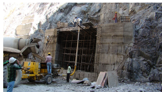
Fig. 1.1 Walls of pump house are supported with the SFRS and rock bolting
