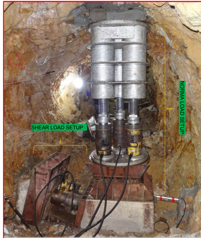
Fig. 3.1 Complete setup of direct Shear test equipment at Wangchhu HEP site
