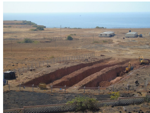
Fig. 4.5 View of three parallel Trenches at stage zero
