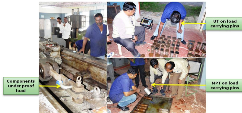
Fig. 9.10. Proof load test and NDT on bucket bows, load carrying pins and D-shackles
