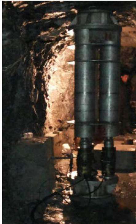
Fig. 3.3 Complete set up of Plate Load equipment at powerhouse cavern of Teesta-IV hydroelectric project
