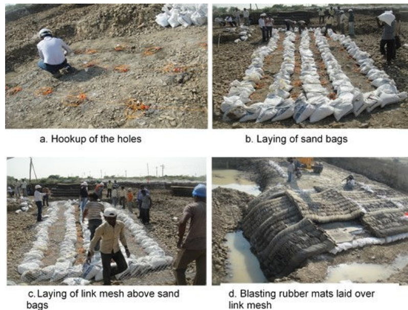
Fig. 6.6 Photographs showing sequence of muffling
