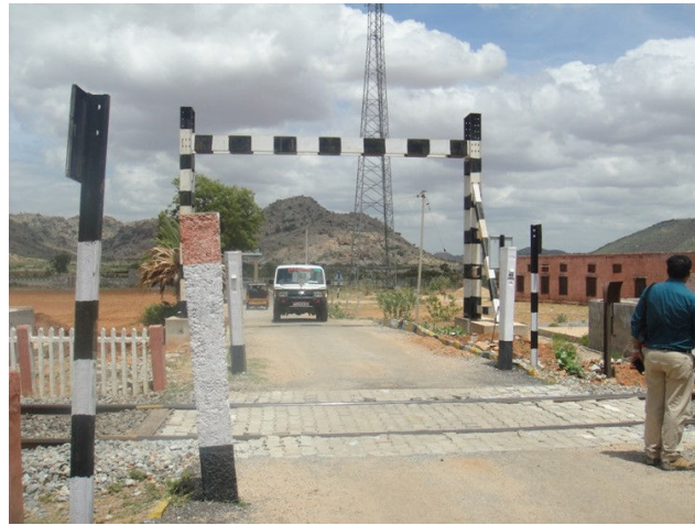
Fig. 6.15 Location of level crossing no 95
