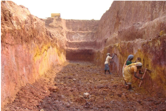
Fig. 4.6 Cleaning of the trench walls to make it ready for mapping
