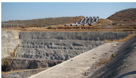
Fig. 1.1 Walls of pump house are supported with the SFRS and rock bolting
