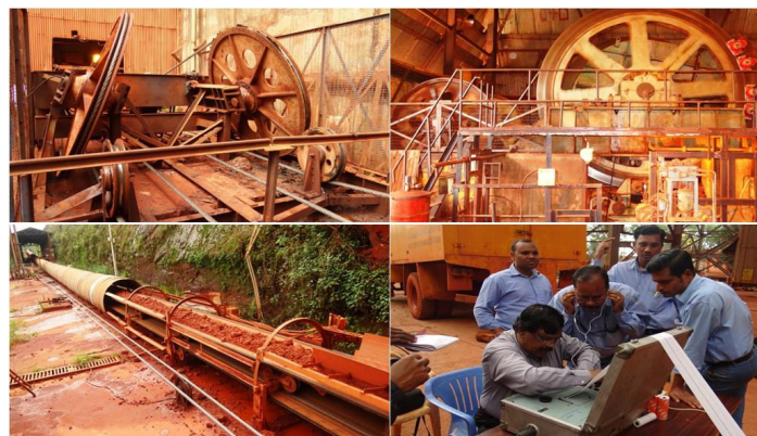
Fig. 9.9 Inspection of cable belt drives
