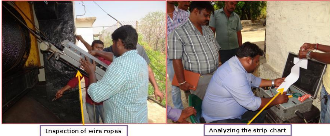
Fig. 8.18 Inspection of wire ropes, M/s KPCL
