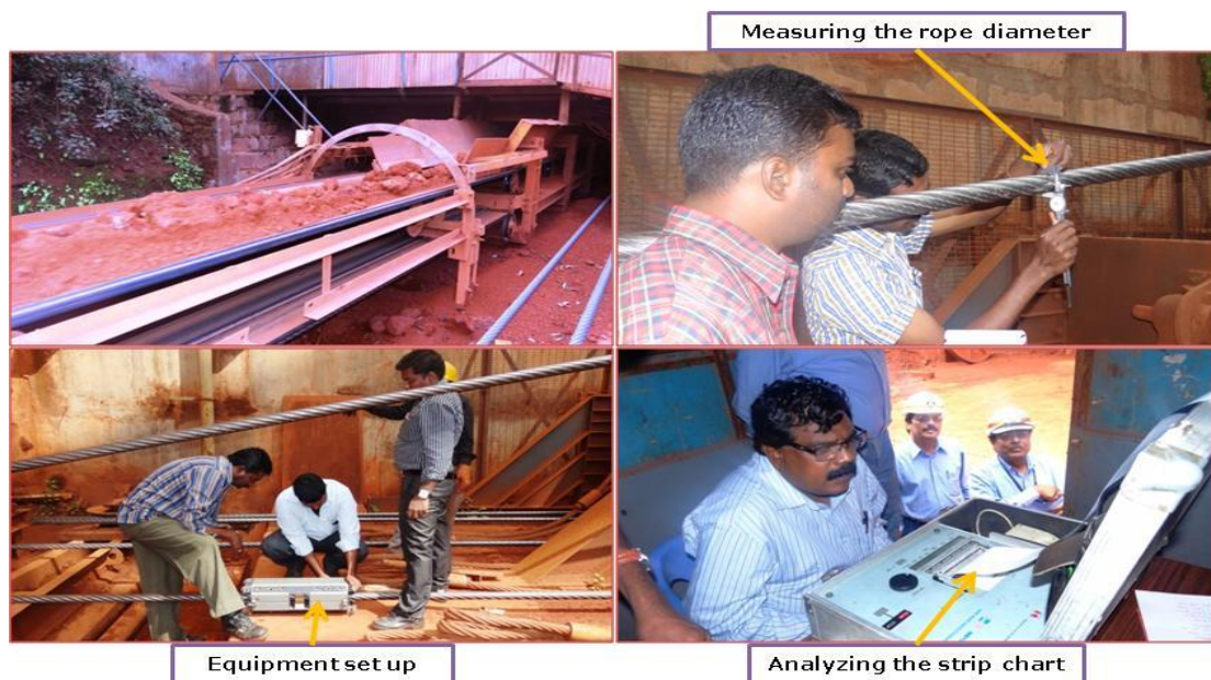
Fig. 8.4 Inspection of cable belt drives, M/s NALCO
