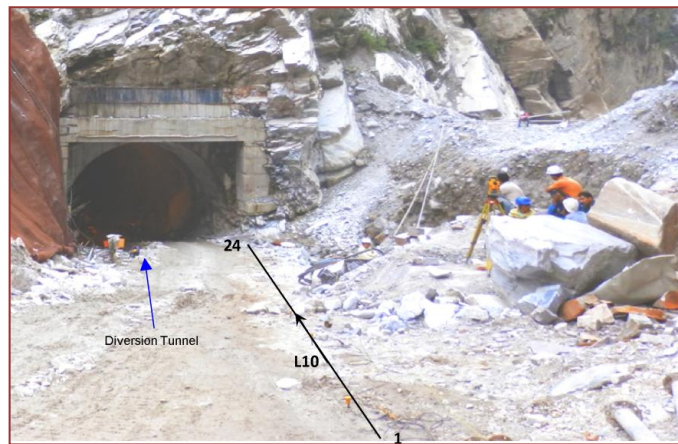
Fig. 2.3 Photograph from diversion tunnel inlet area showing survey lines (L10)
