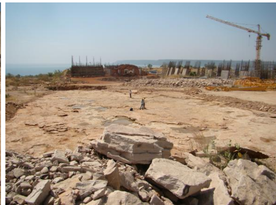
Fig. 1.9: Purplish - yellowish brown quartzitic sandstones exposed at CWPH-7 foundation level
