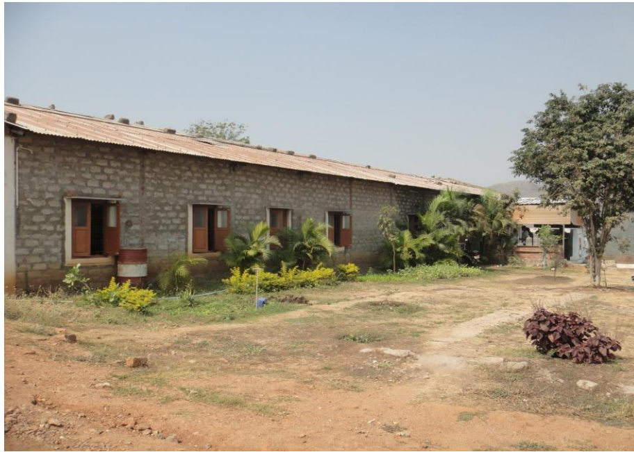
Fig. 6.8 Monitoring of ground vibration and air overpressure in front of police camp
