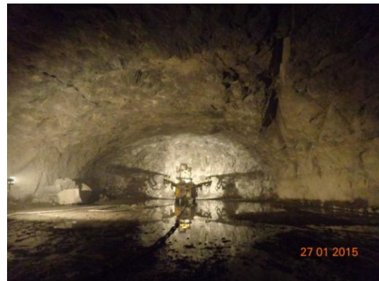
Fig. 1.3: End wall of pump house at chainage 210.6 m
