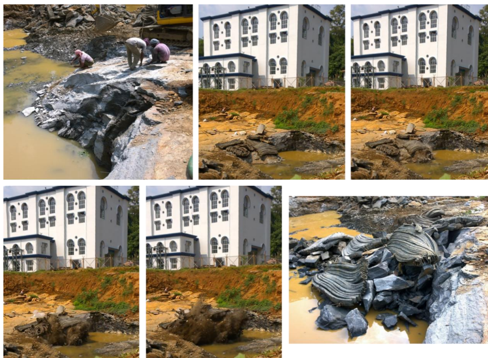
Fig 6.3 Blasting close to existing powerhouses
