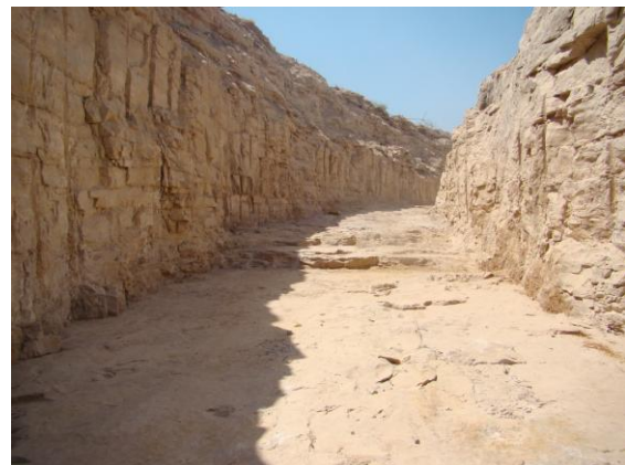
Fig. 1.7: Purplish/yellowish brown quartzitic sandstone exposed at tower foundation level
