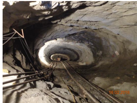
Fig. 1.5: View of excavated escape tunnel from Medaram side
