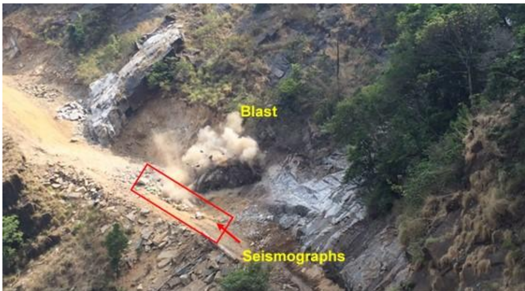
Fig. 6.1 Blasting adjacent to buried petroleum pipeline
