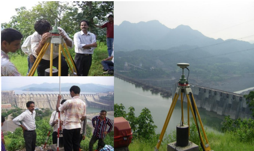
Fig. 5.4 Control points establishment at SSNNL Dam
