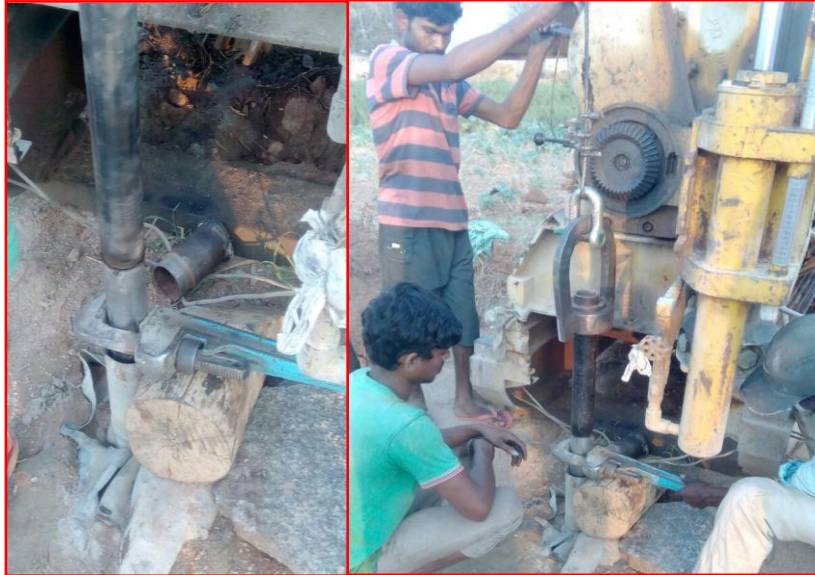
Fig. 3.5 Lowering of hydraulic fracture equipment with NQ rods
