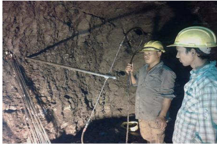
Fig. 10: Hydraulic fracture test under progress at BH 1 Vishnugad Pipalkoti H.E. Project
