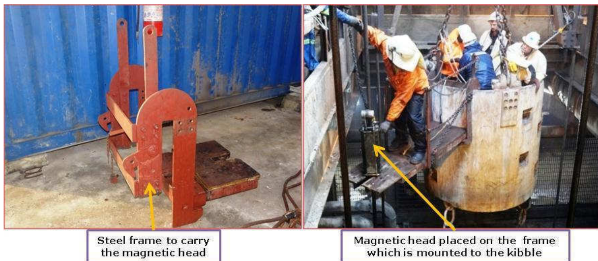
Fig. 62: Testing of stage winder ropes, M/s SSM.
