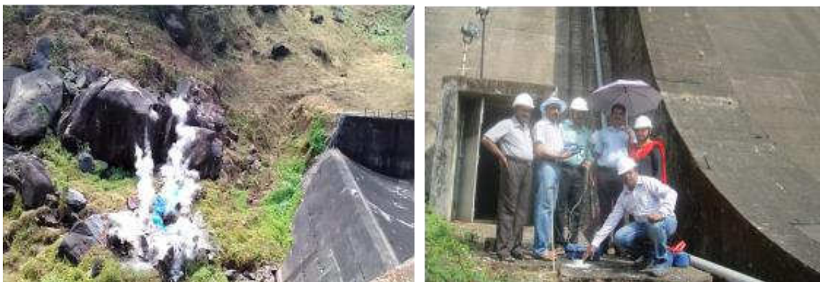
Fig. 26: Blasting close to dam structures and monitoring of ground vibration
