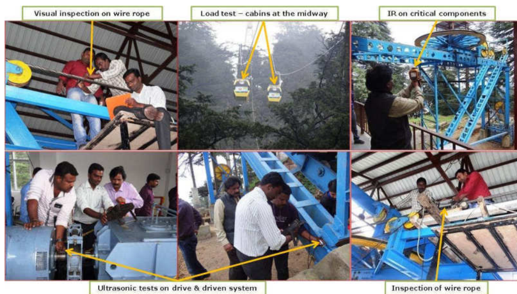
Fig. 66: NDT on aerial ropeway system, M/s JIL.
