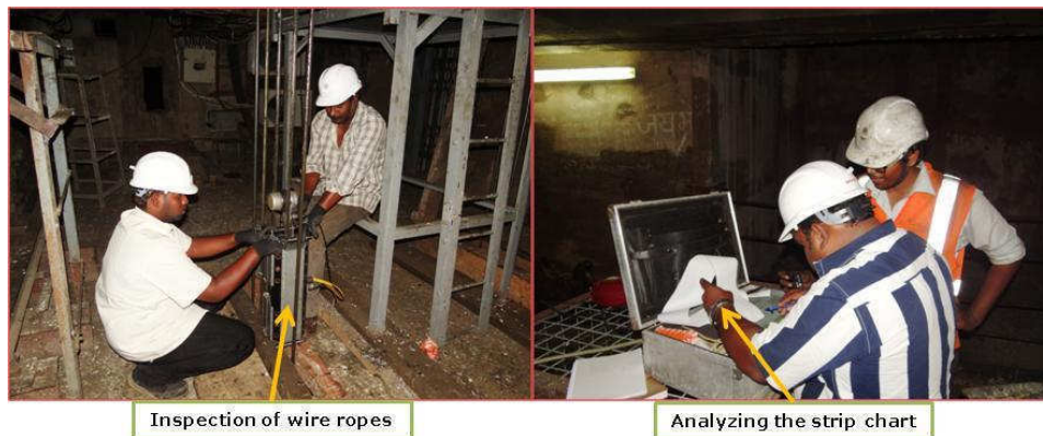
Fig. 57: Inspection of wire ropes, Rajpura Dariba mines, M/s HZL.
