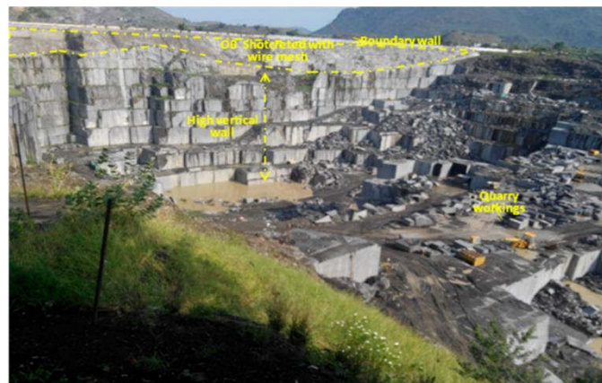
Fig. 21: A view of overburden supported with shotcrete in Pallava granite quarry
