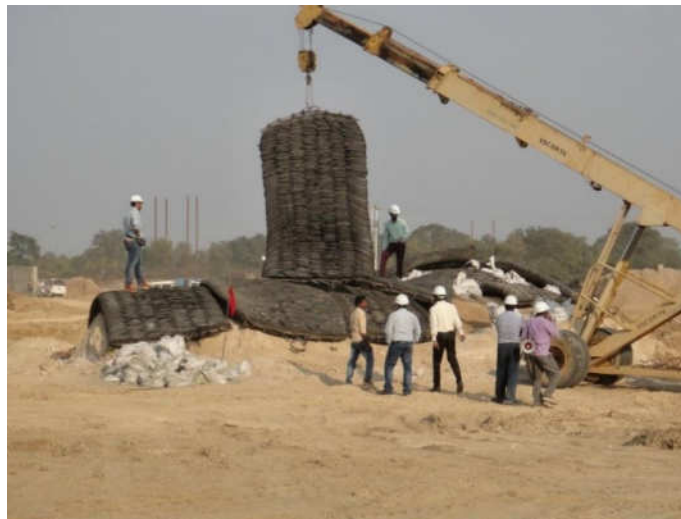
Fig. 32: Laying of blasting rubber mats over link mesh for controlled blasting
