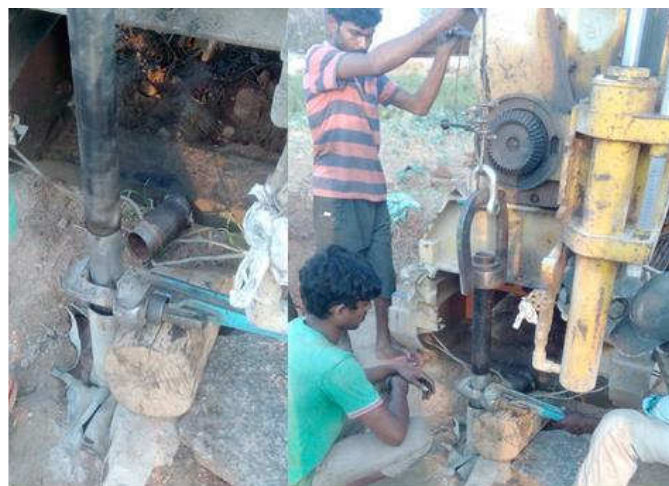
Fig. 8: Lowering of hydraulic fracture equipment at PCILS, package no 11
