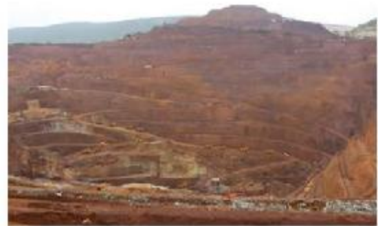
Aerial view of the Kaliapani Chromite Mine showing dumps on its boundary.
