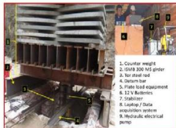
Field setup for measuring of safe bearing capacity
