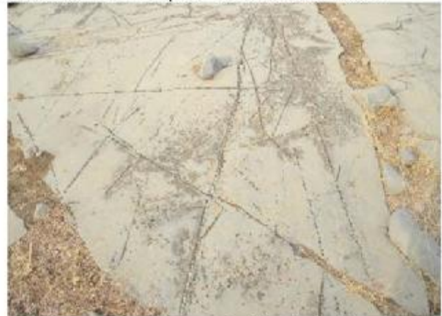
Holes developed along the joint in the limestone
