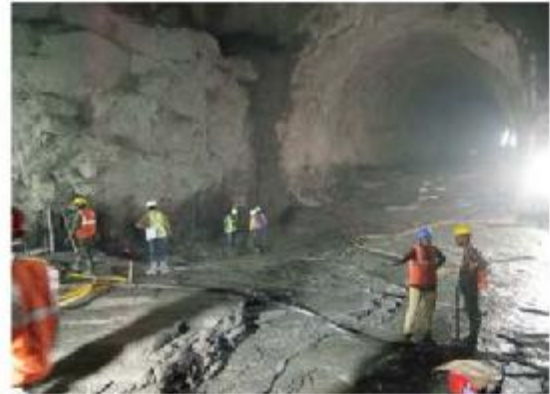
Cleaning of the pump pit-1 foundation area for engineering geological mapping
