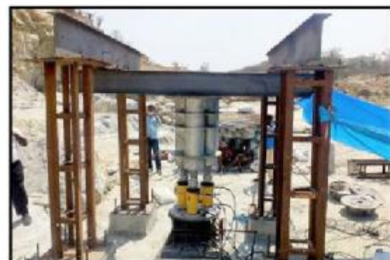
Direct shear test being carried out at the Yargol dam project
