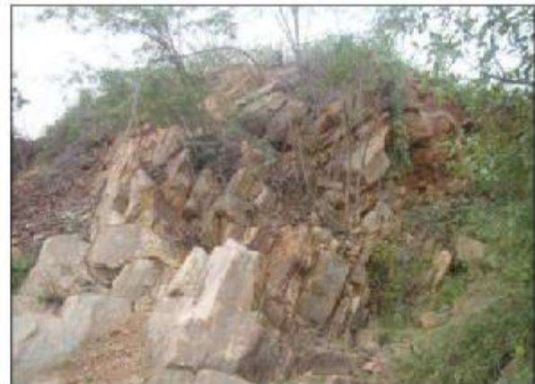
West dipping fault observed in the direction of lineament N 8.
