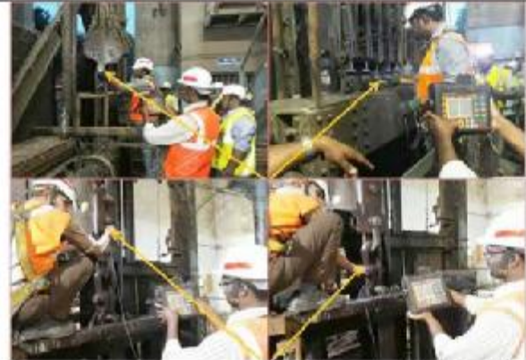
NDT on suspension gear parts, Rajpura Dariba Mines
