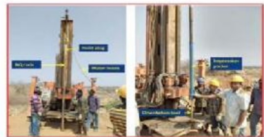
Lowering of hydraulic fracturing equipment with NQ rods
