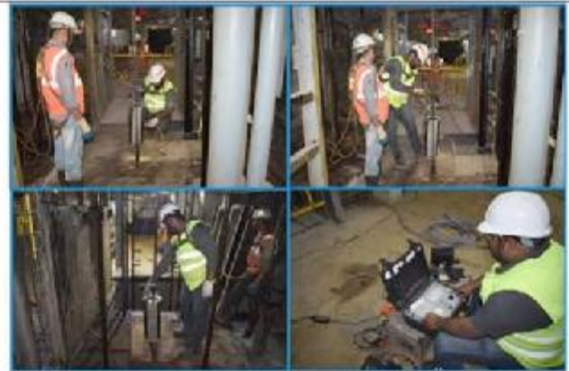
Inspection of wire ropes, Zawar group of mines, HZL
