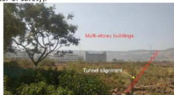
Location of various civil structures with reference to the proposed twin-tunnel alignment
