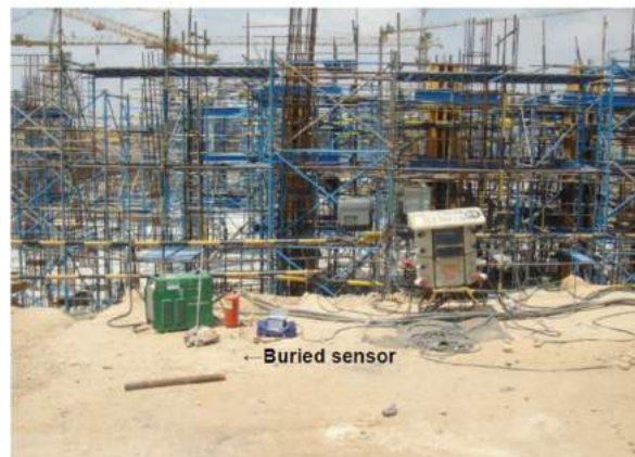
Monitoring blast vibration 6m before TB3
