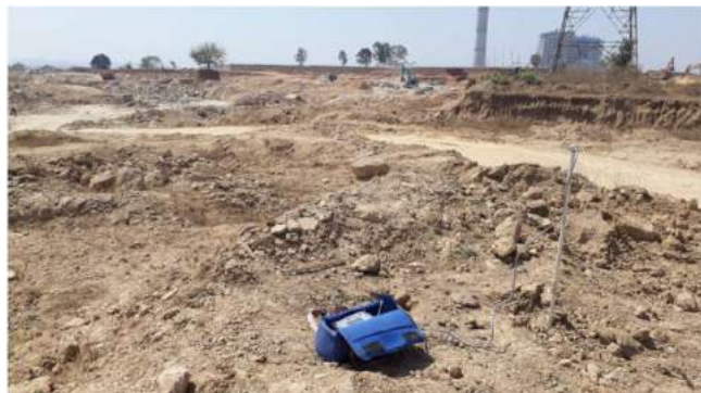
Monitoring ground and air overpressure towards Darlipalli village
