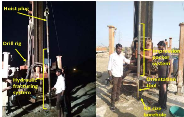
Lowering of hydraulic fracturing equipment with NQ rods
