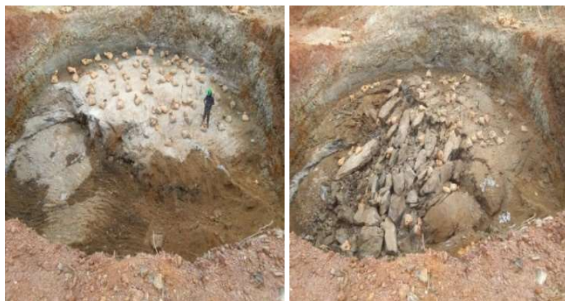
Site before and after blast photographs taken at surge shaft
