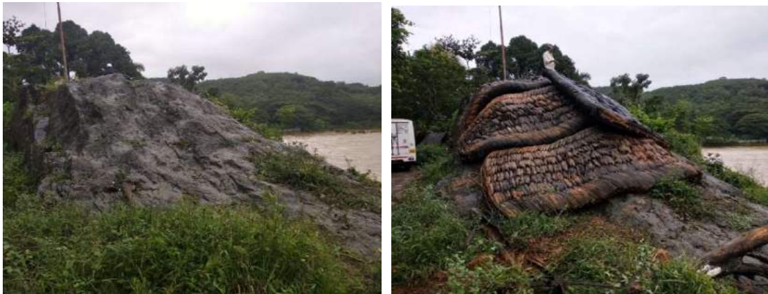
Blast location showing before and after muffling with rubber mat
