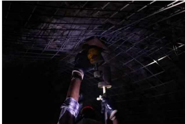
Rock bolt anchorage testing in the Mine
