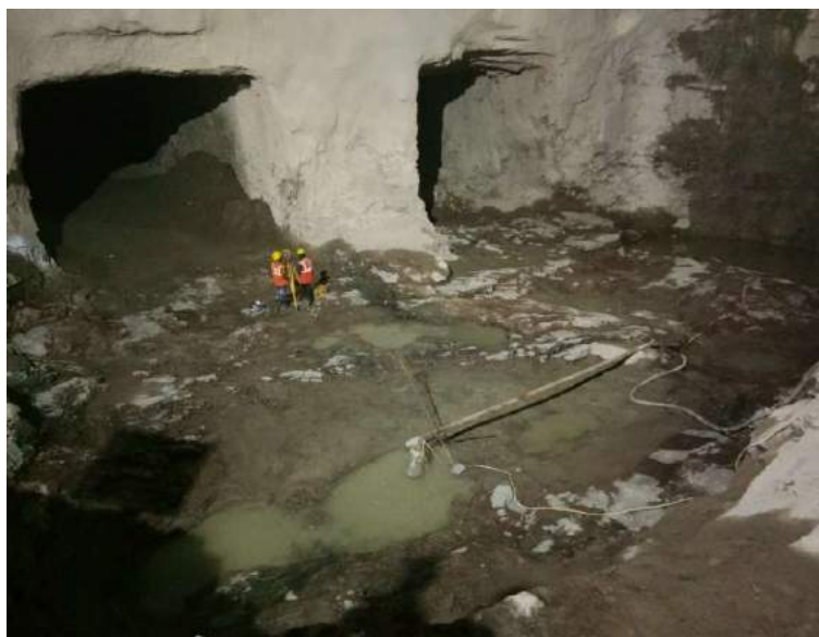
Foundation of Pump Pit-land 2
