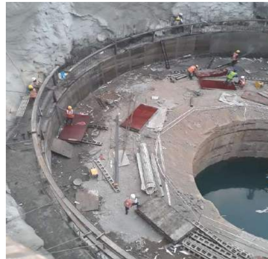
Excavation of Circular Pump-house
