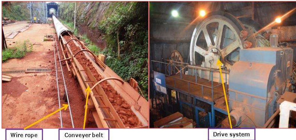
Inspection of cable belt drive ropes, M/s NALCO
