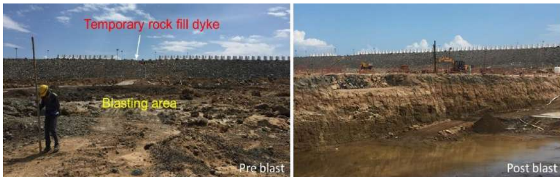
Controlled blasting adjacent to temporary rock fill dyke
