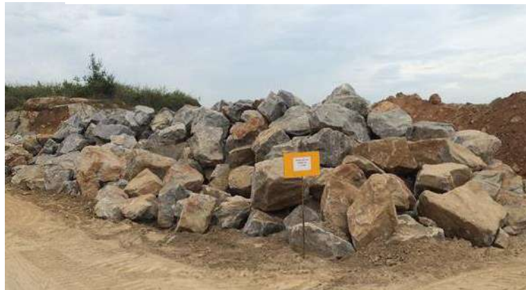
Required armour stone of 6MT
