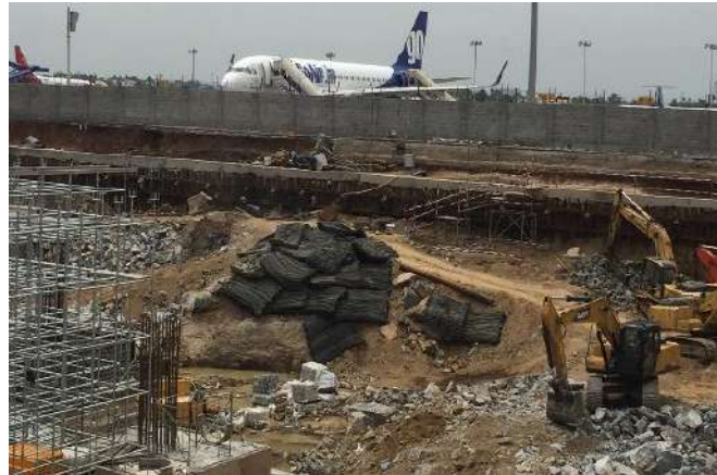
Controlled blasting in an operating airport for expansion work
