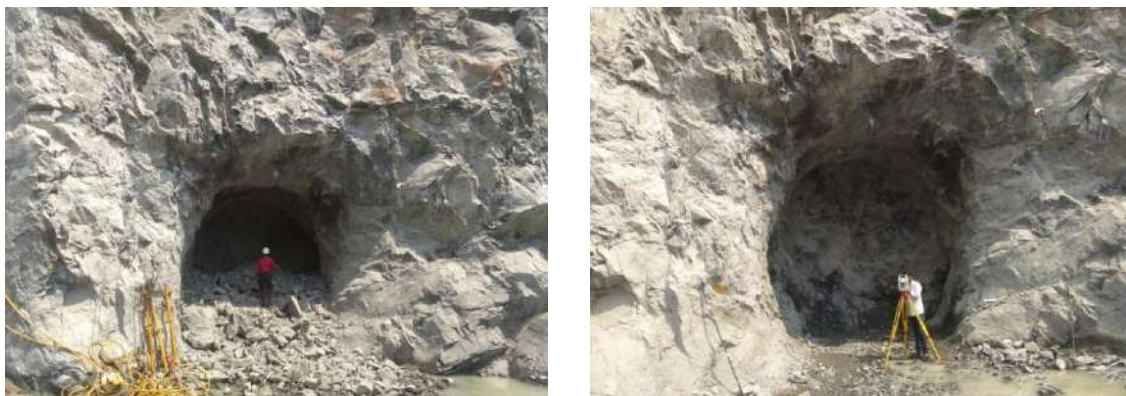
Photograph show post blast and neat profile in Penstock 2
