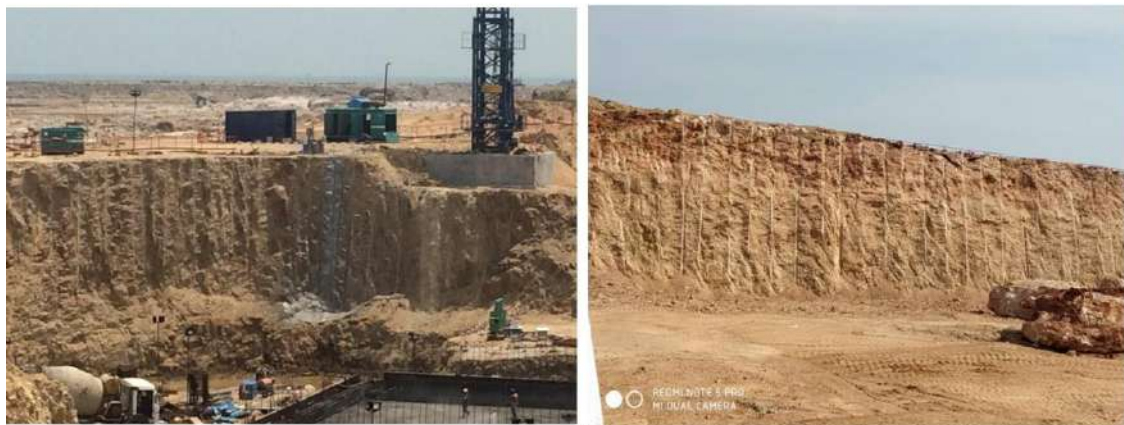
Controlled blasting close to green concrete
