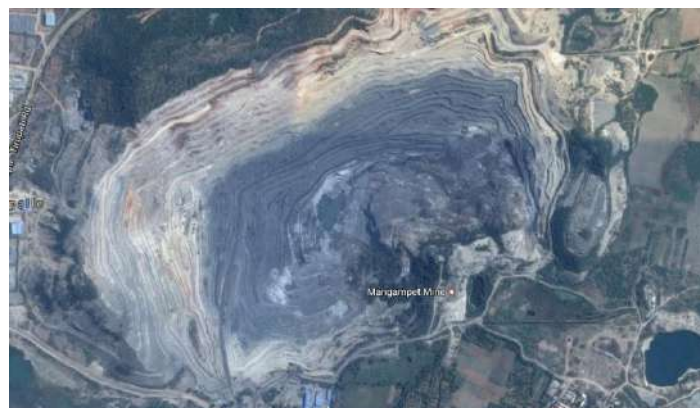
Satellite image of the Dolomite Project
