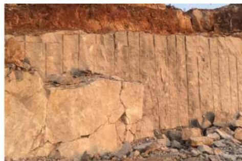
Slope obtained as a result of presplit blast design
