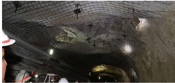
Wiremesh installation in the old drives of Zawarmala
