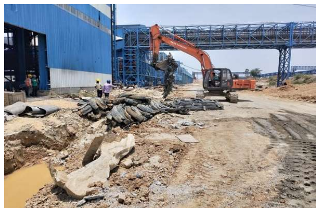
Controlled blasting adjacent to the structures
