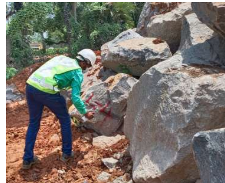
Marking of armour rock at stock pile.
