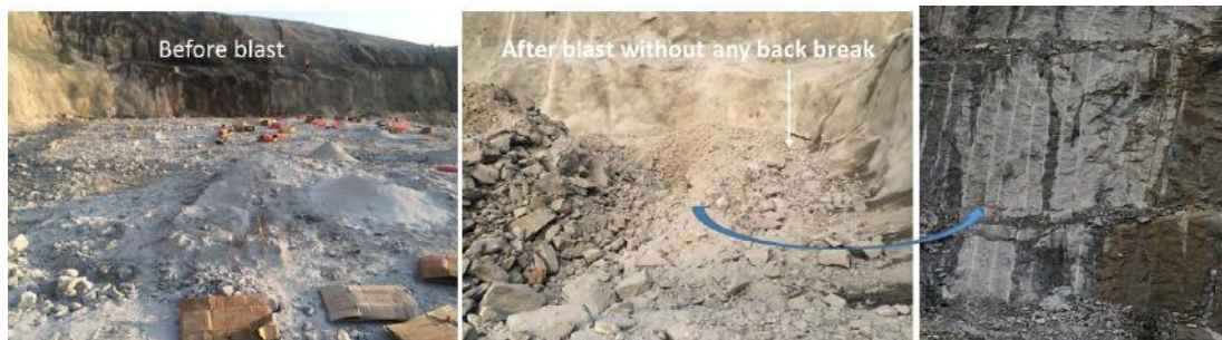
Slope obtained as a result of presplit blast design
