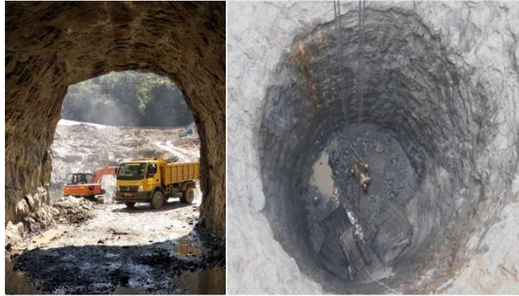
View of Head Race Tunnel (left) and surge shaft (right) excavation
