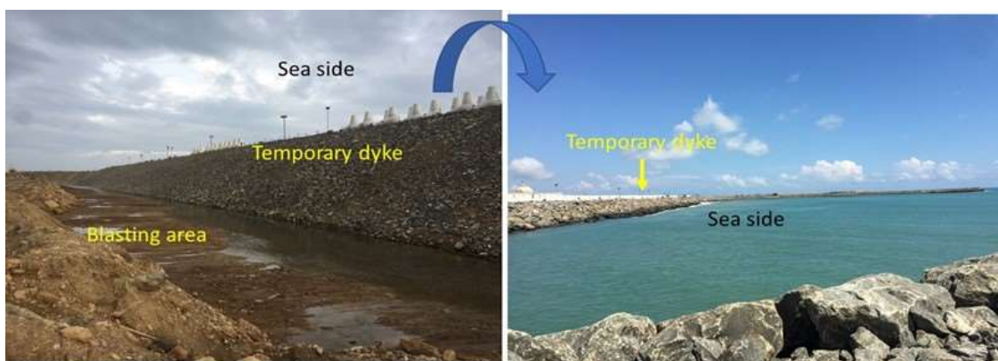
Controlled blasting close to a temporary dyke
