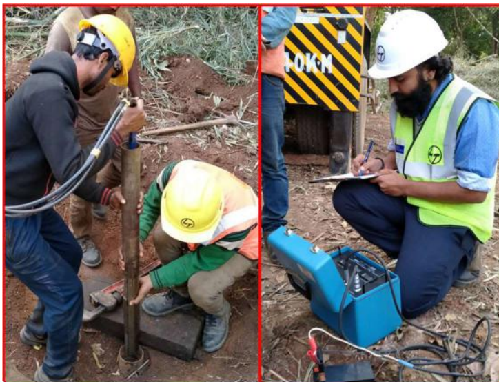
Goodman Jack test in progress at test location SS1
