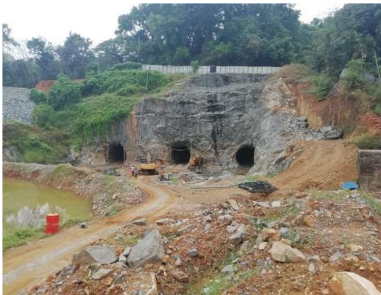
Excavation of 3 tunnels near Pazhassi Sagar barrage
