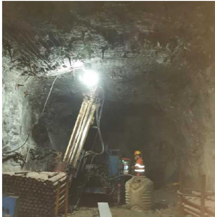
Hydraulic fracturing test at Zawar mines (HZL)
