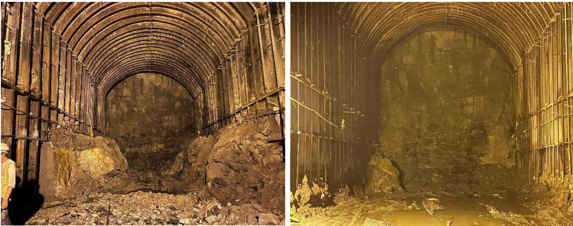
Final benching excavation in AST-N1a at RD 110
