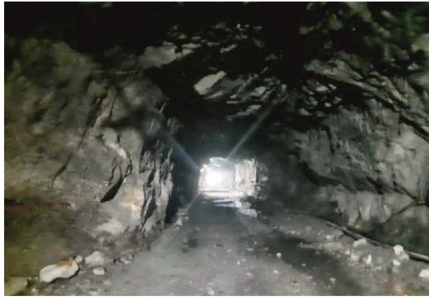
Geotechnical mapping at drive of Malanjkhanda Underground Copper Mine
