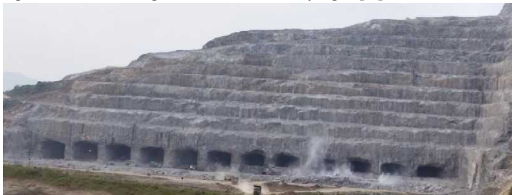
Panoramic view of all pressure tunnels from the intake site of PHEP
