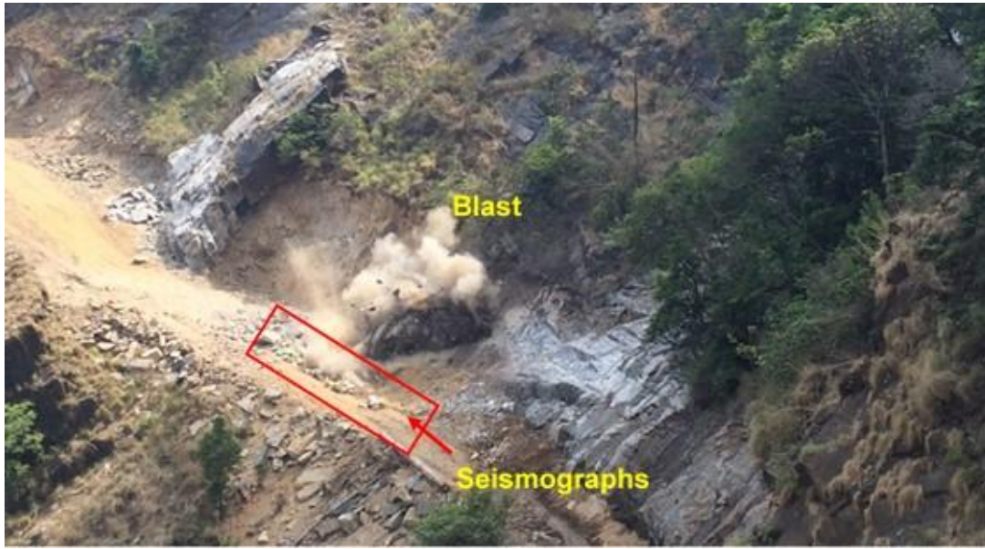
Fig. 6.1 Blasting adjacent to buried petroleum pipeline
