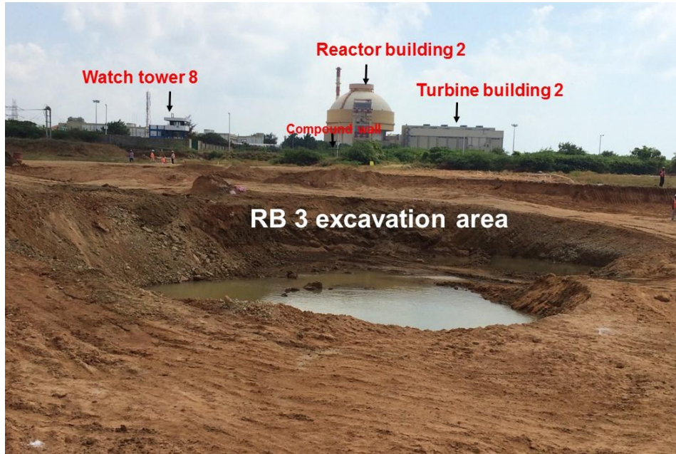
Fig. 6.7 View of proposed excavation site RB 3 and commissioned unit 1&2
