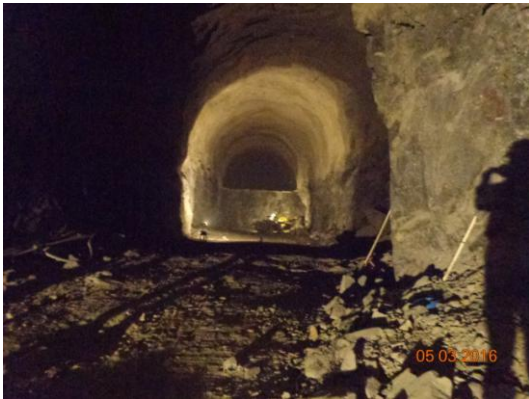
Fig. 1.4: Bench excavation under progress in the transformer cavern
