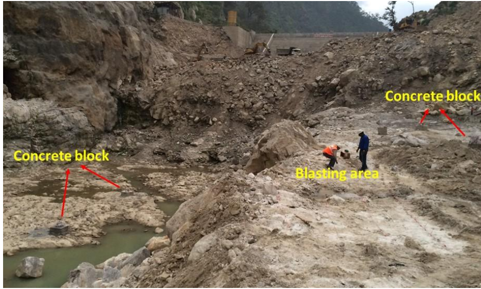
Fig. 6.6 Location of concrete blocks casted and experimental blast locations
