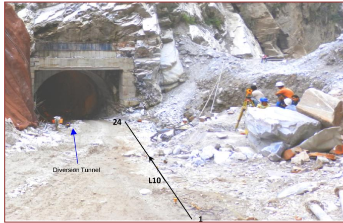
Fig. 2.3 Photograph from diversion tunnel inlet area showing survey lines (L10)
