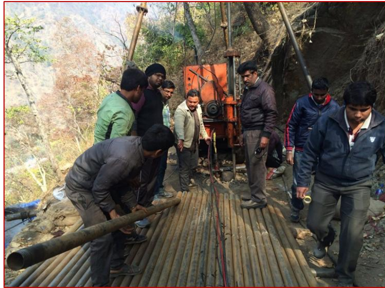
Fig. 3.3 Lowering of hydraulic fracture equipment with NQ rods
