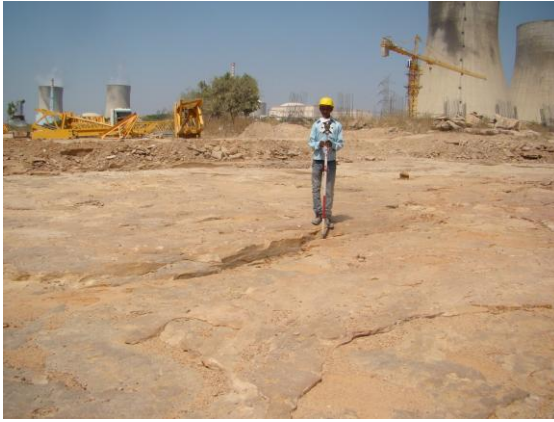
Fig. 1.8: Collection of data after cleaning of the CWPH-7 foundation
