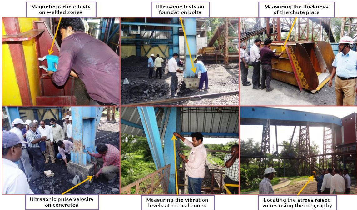
Fig. 8.7 NDT on steel structures of Ramkrishnapur Coal Handling Plant (CHP), Mandamarri Area. M/s SCCL
