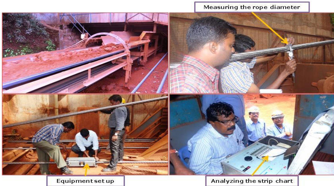
Fig. 8.4 Inspection of cable belt drives, M/s NALCO
