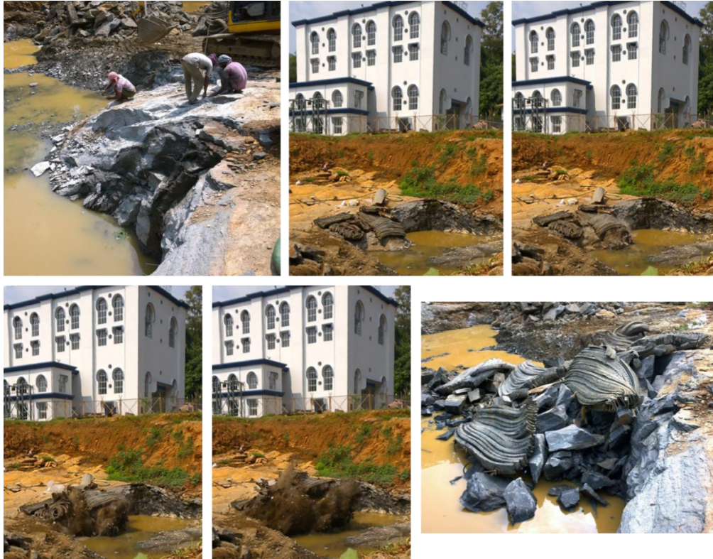
Fig 6.3 Blasting close to existing powerhouses
