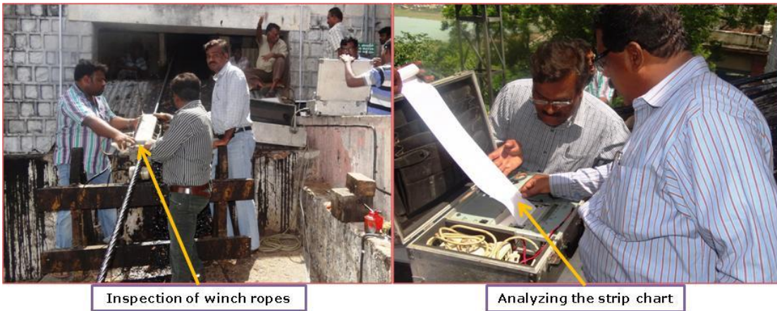
Fig. 8.14 Inspection of winch ropes, M/s ADST
