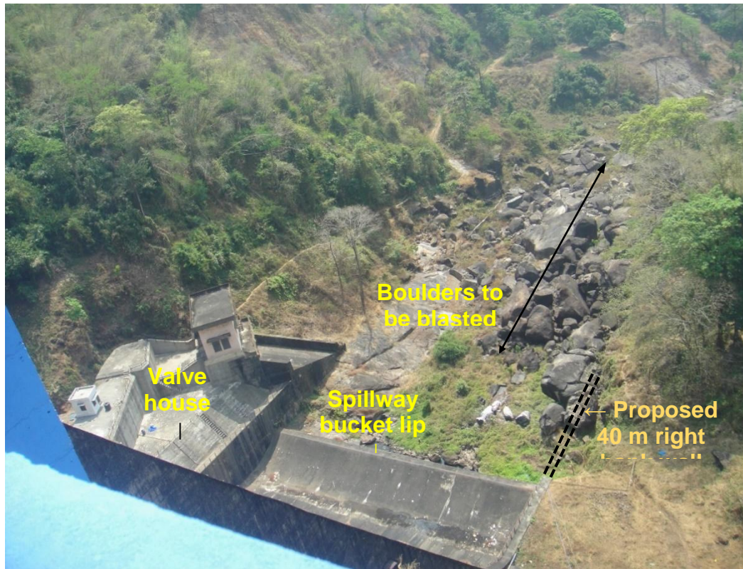
Fig. 6.12 Quantity of boulders to be blasted close to dam structures
