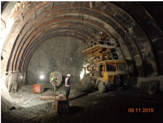
Fig. 1.2: Rib erection work under progress at chainage 3023 m in RMT upstream
