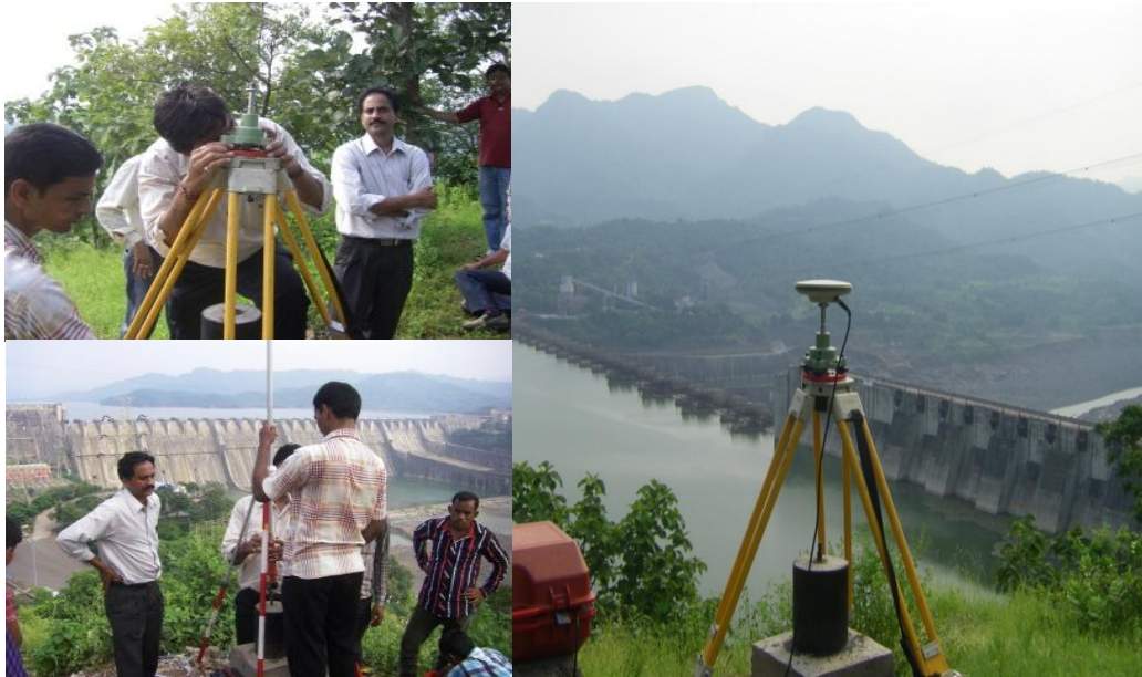
Fig. 5.4 Control points establishment at SSNNL Dam
