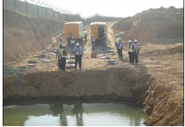
Preparation of charging of holes for bench blasting
