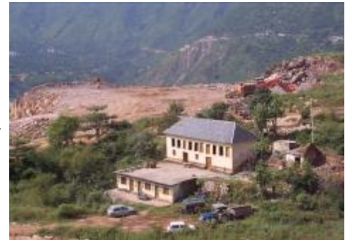
Controlled blasting experiment near existing structure at Koladam Hydel Project site
