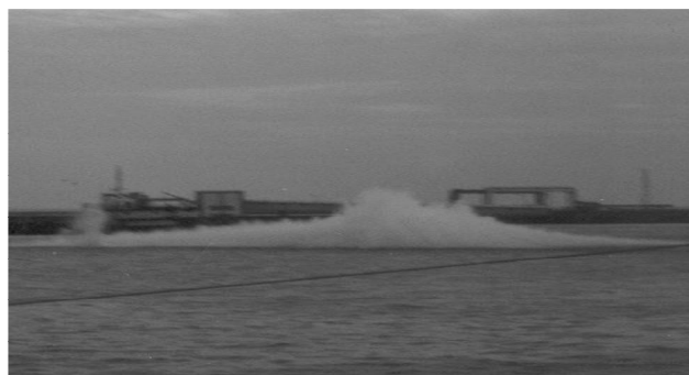
Fig. 10. Underwater blasting in progress
