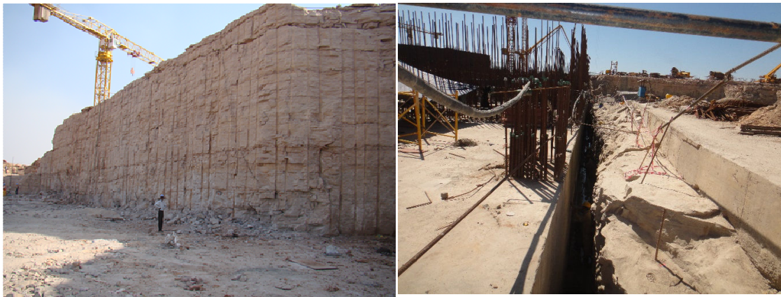
Fig. 6. Pre-split blast wall and the subsequent civil constructions of the nuclear plant
