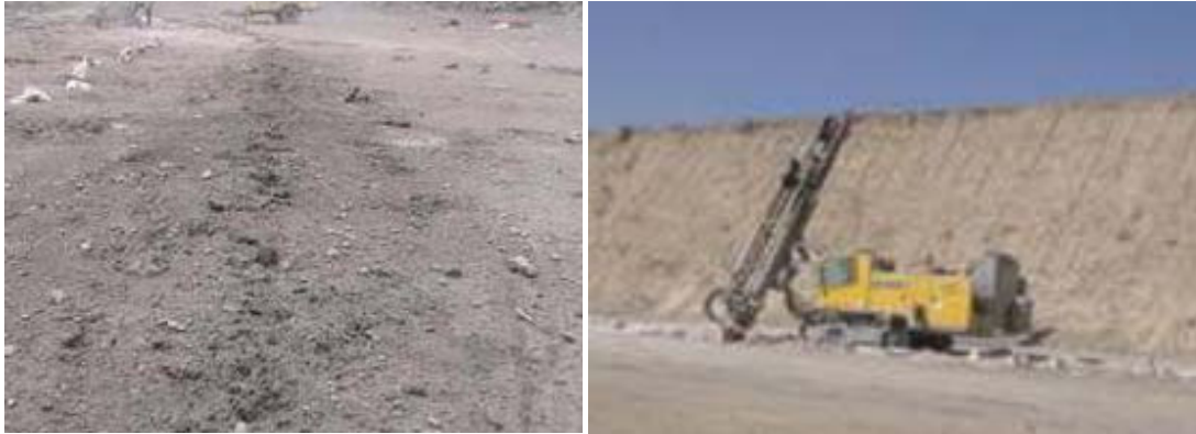
Fig. 5. Pre-split blasting at Rampura Agucha mine
