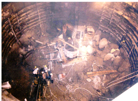
Fig. 9. Full face blasting of 16 m dia surge shaft
