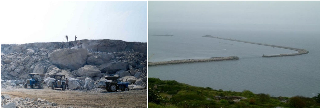
Fig. 11. Blasted armour rock and the finished break water on the sea
