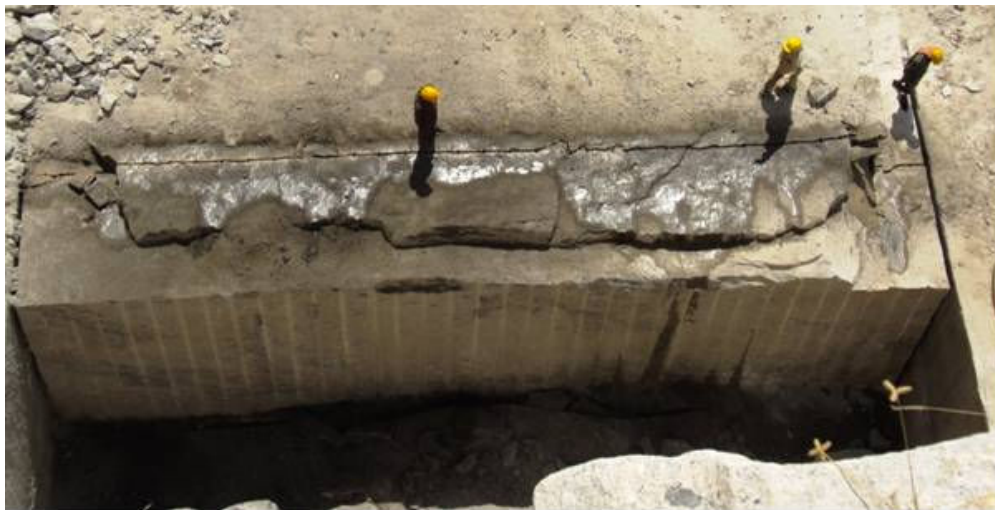
Hole to hole splitting with detonating cord
