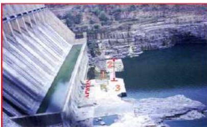
Cavity mapping in the apron of Srisailem dam using Seismic survey
