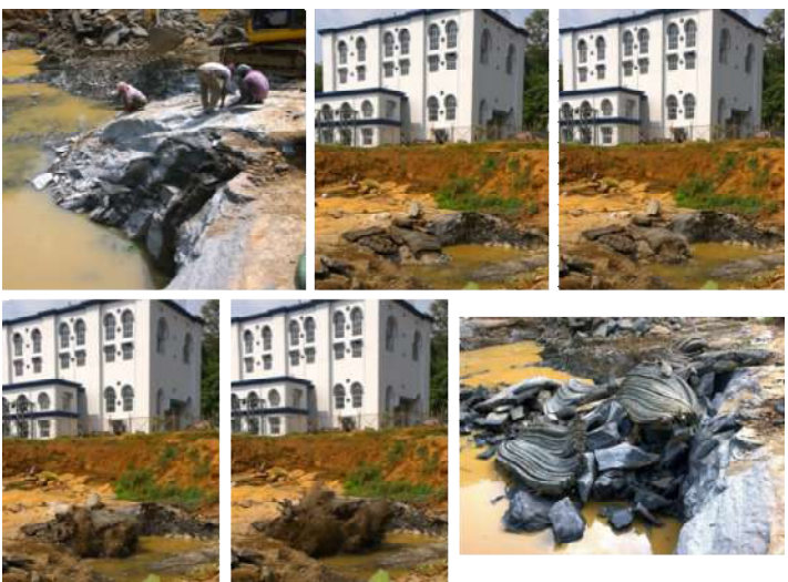
Blasting close to operating powerhouse, KSEB
