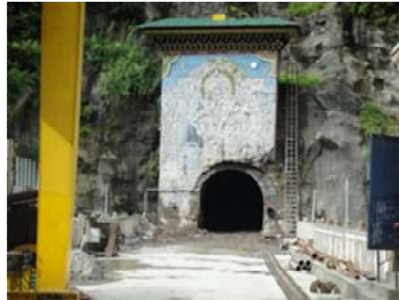
Successful excavation of tunnel at left bank abutment, Tala concrete dam, Bhutan
