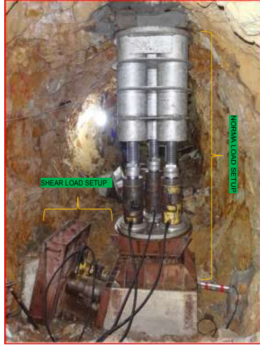
In-situ Direct Shear tests (inside the tunnel) at Dibang H.E. Project, Arunachal Pradesh
