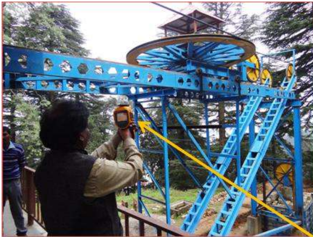
Infrared Thermography studies on an Aerial Rope Way system, Shimla
