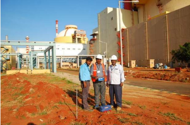
Blast monitoring adjacent to reactor building, KKNPP, Kudankulam, Tamilnadu
