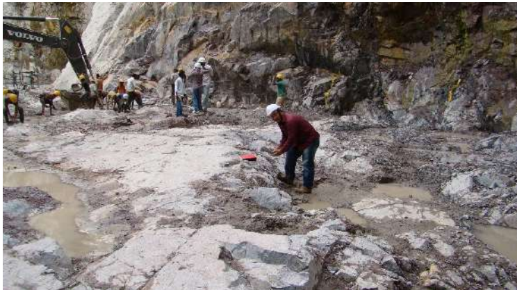
Collection of engineering geological data from surge pool foundation
