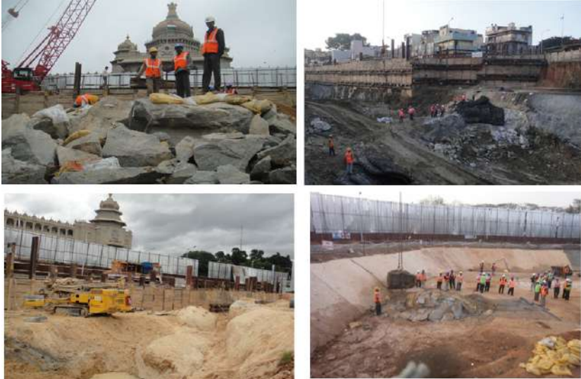
Controlled blasting at different underground stations, BMRL
