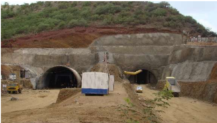
Excavation of tunnel portals, back and side slopes
