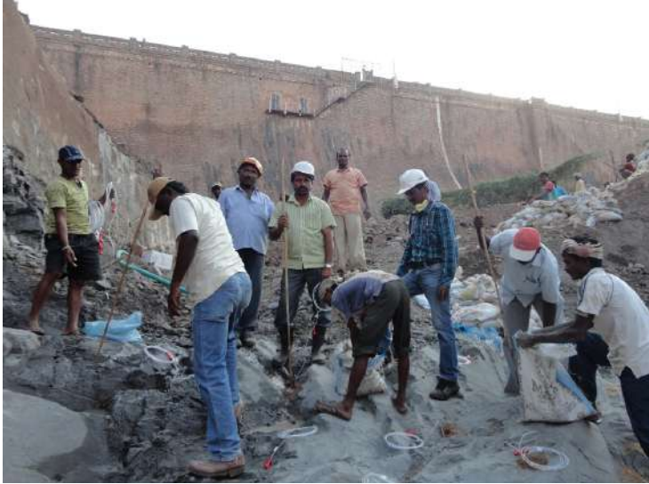
Technical guidance on controlled blasting procedure close to Tungabhadra masonry dam, Karnataka
