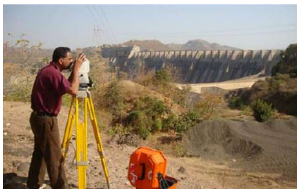
Geodetic monitoring of Sardar Sarovar Dam.
